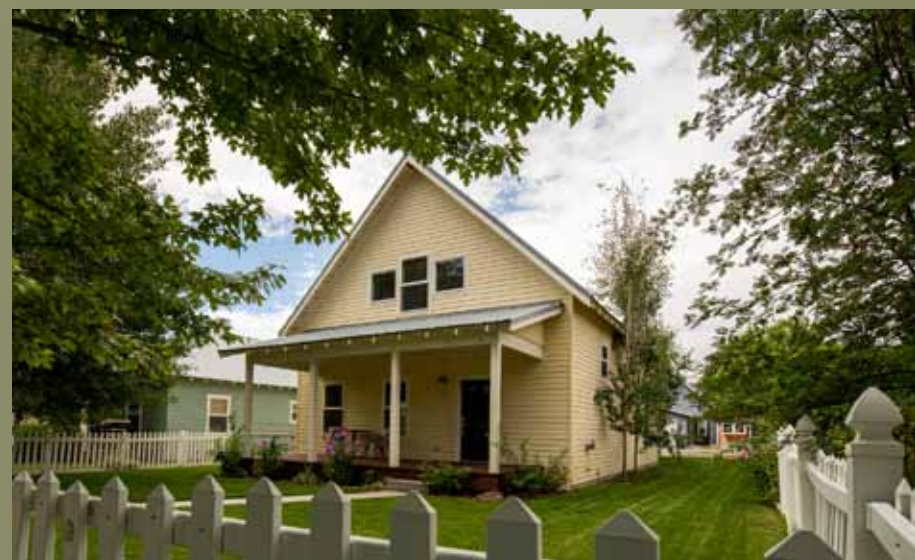
Photo Credit: Josh Wells
